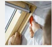
The vapour barrier helps prevent the build-up of condensation in the roof construction. Ideal for making your installation air tight
