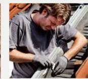
An underfelt collar ensures a weather tight seal and eliminates cold bridges. Again, this helps you to meet building regulations.
